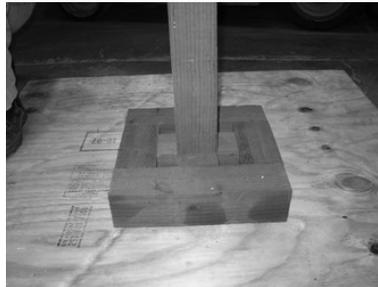
1) Install blocking around load bearing support (typically pressure treated wood). Blocking should be made from pressure treated wood, and must be the same size as the inside of the pedestal/newel.
