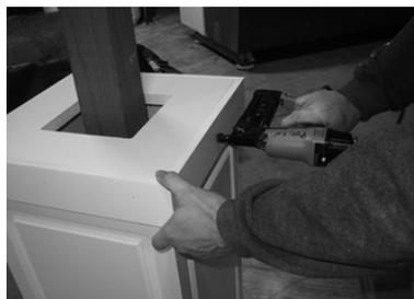
10) Apply glue to backs and mitered edges of cap moldings, then assemble to shaft below top platform with pin-nails. (Mouldings, panels, trim, and top platforms may vary from photos depending on product styles.)
