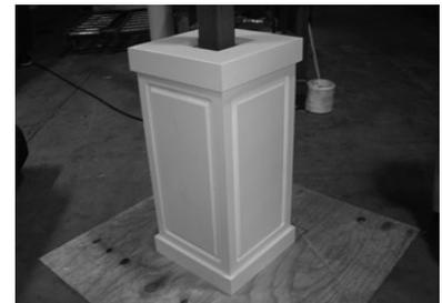
11) Caulk all seams, fill all nail holes, and clean surfaces with cleaner recommended by paint manufacturer. Finish with two coats of acrylic latex paint.
