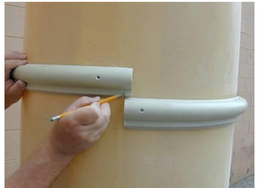
12) Hold the untrimmed neck ring half in position so it can be marked for proper fit.
