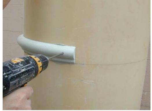
10) After installing the two screws in the center of the part, install the last two screws at the ends of the part. This sequence will result in a better fit.
