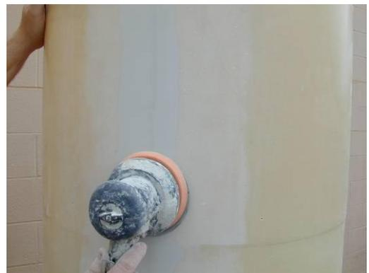
6) Sand cured body filler. For best results, use care when sanding to maintain an even radius. Finish with 120 grit paper.
