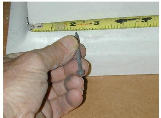
Use long enough screws to secure to plywood on the inside of the other cap or base half.
