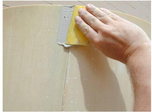
4) Mix body filler (not supplied) according to manufacture's instructions and apply to joint. Make joint wide enough to make a smooth radius.
