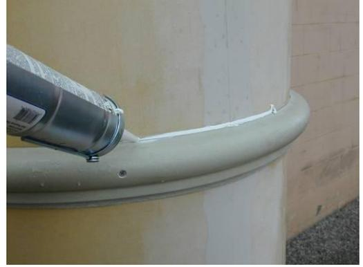
15) Apply a bead of good paintable exterior chalk at the top and bottom joint where the neck ring joins the column. Smooth bead for proper appearance.
