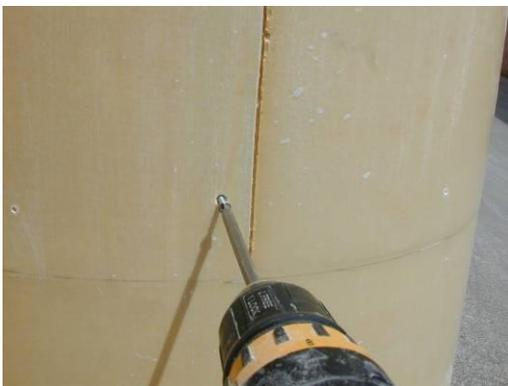
3) Countersink and install screws at each reinforced rib, using provided self-drilling 1" screws.
