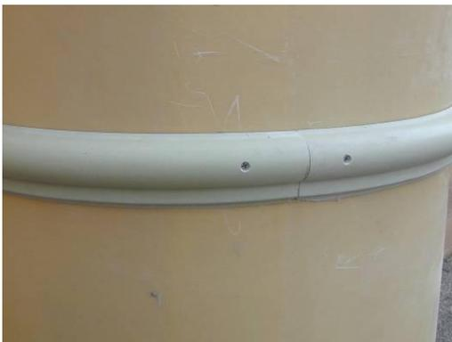
14) Check fit and install the second neck ring half with adhesive and screws.
