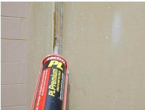
2) After trimming column sections to fit, apply adhesive to joints.
