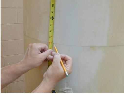
7) Draw a line around the top of the column 16" down from the top of the column. This is the suggested location for the bottom of the neck ring.
