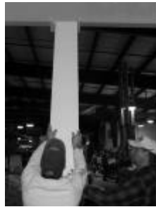
14) Assemble final panel to column using E-Z lock joint
