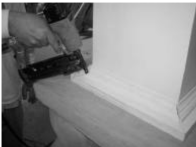
19) Apply adhesive to moulding and pin-nail into place.
