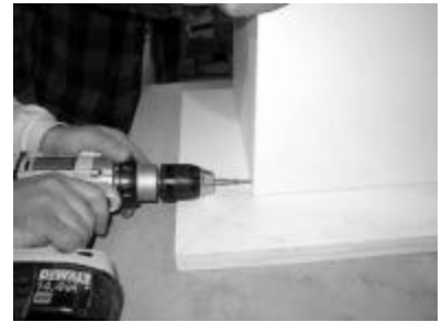
15) Screw or nail final panel to secure
